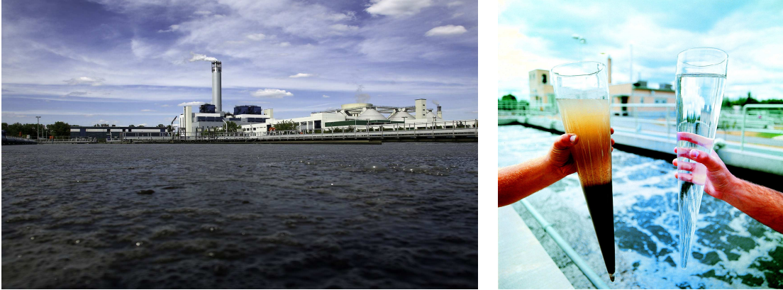
Figure 2.3: Waste water treatment plant in Ruhleben (modernized by the German subsidiary) and comparison of a water sample before and after filtration. Ruhleben is the largest and most important waste water treatment plant in the greater Berlin area and processes 240,000 cubic meters of waste water daily.
